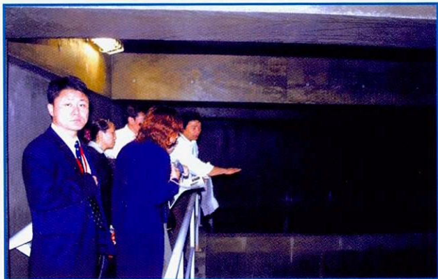
Storm water sedimentation tank located under Yokkaichi Dome
