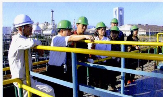
Kasumi Kyodo Jigyo Co., Ltd.: On-site training at the wastewater treatment plant
