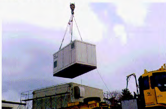
Photo 1: LPG fueled fuel cell power plant
