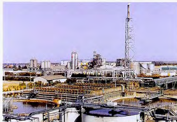
Wastewater treatment facility
