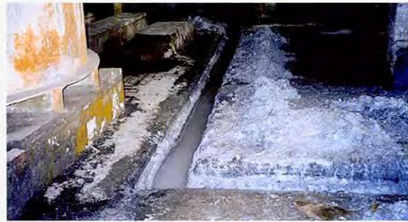
Wastewater drainage in the fertilizer factory
