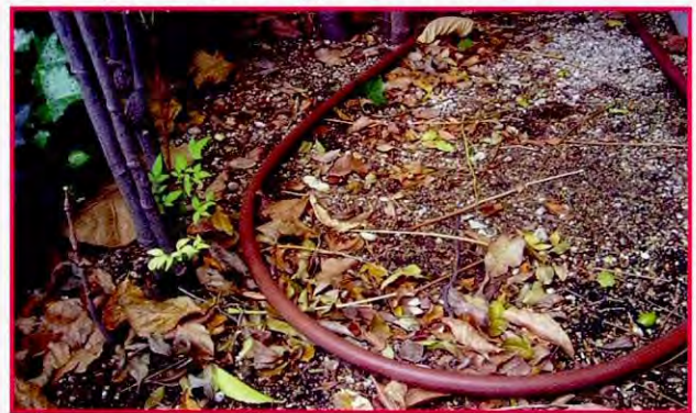
Water being sprinkled at the rooftop garden of Namba Parks (Water drips out of holes in the hose as watering begins drop by drop when the rain detector fails to detect rainfall for an extended period of time.)
