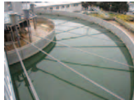
Frozen food processing plant of "A" company
