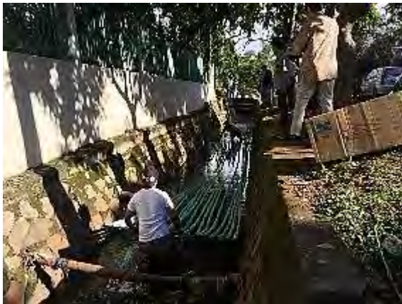
Installation example in Jakarta City Installation work completed in 1 day
