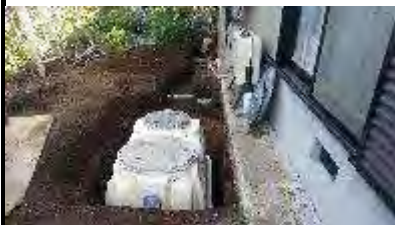
General way of installing jokaso
